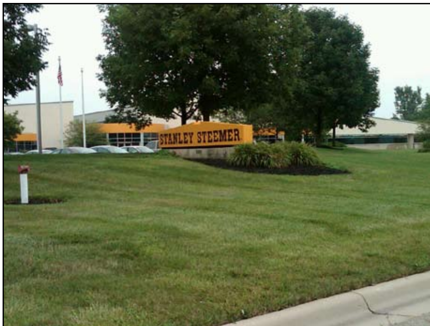
The Dublin facility will cut in half the $250,000 cost to replace AC units.
