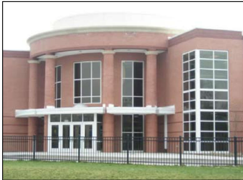
Wellington School switched to energy-efficient gas-fired heat.
